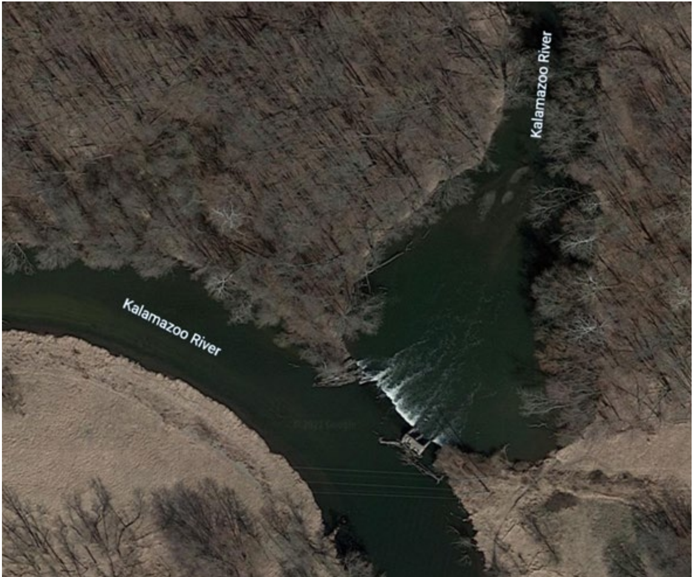
A.2. Diversion Dam, South of City Limits
