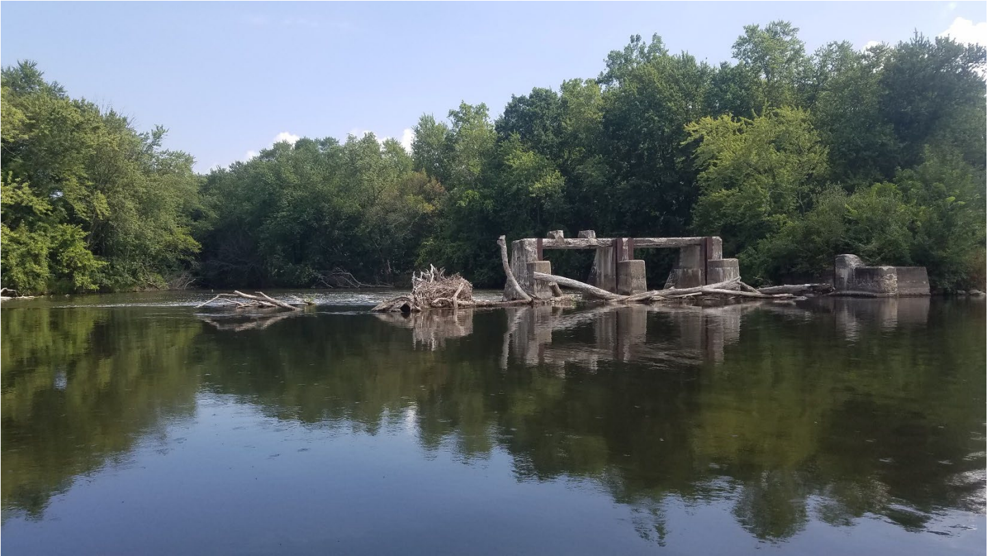
A.4. Plainwell Diversion Dam 2 (primary).
