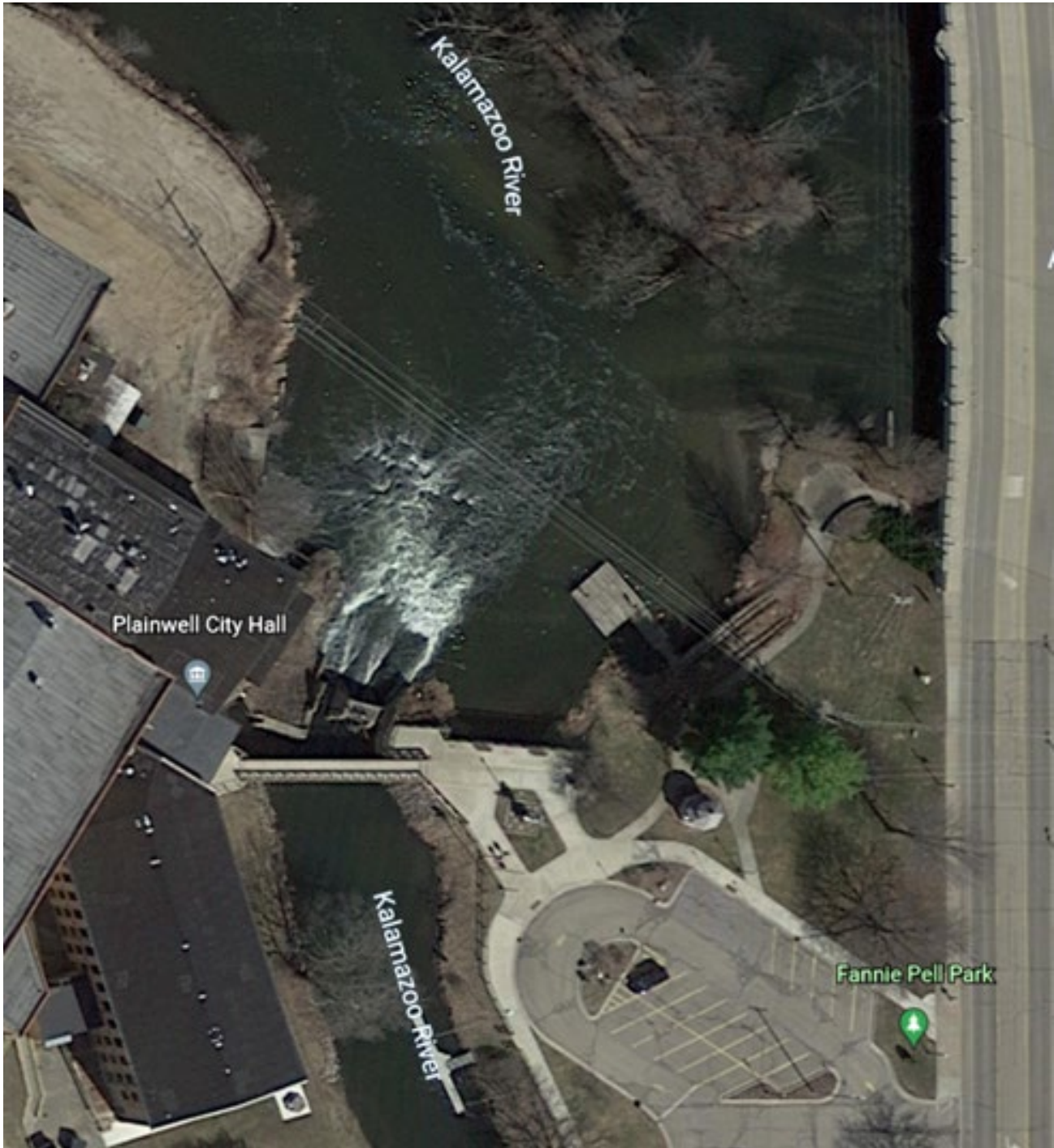
A.7. Downstream – Mill Race, Spillway Plainwell City
