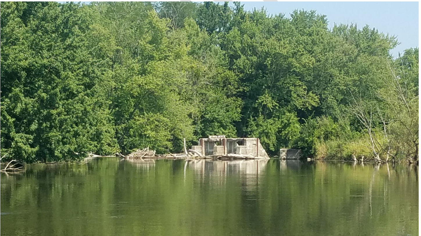
A.5. Plainwell Diversion Dam 2 (primary).
