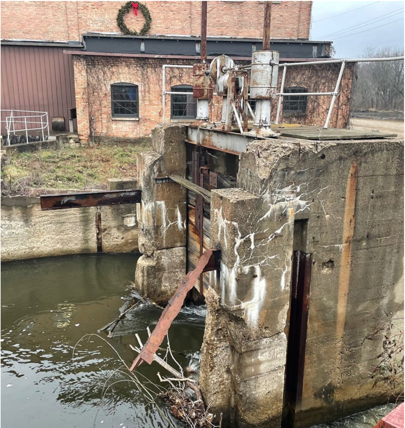
A.8. Concrete remnants in front of City Hall
