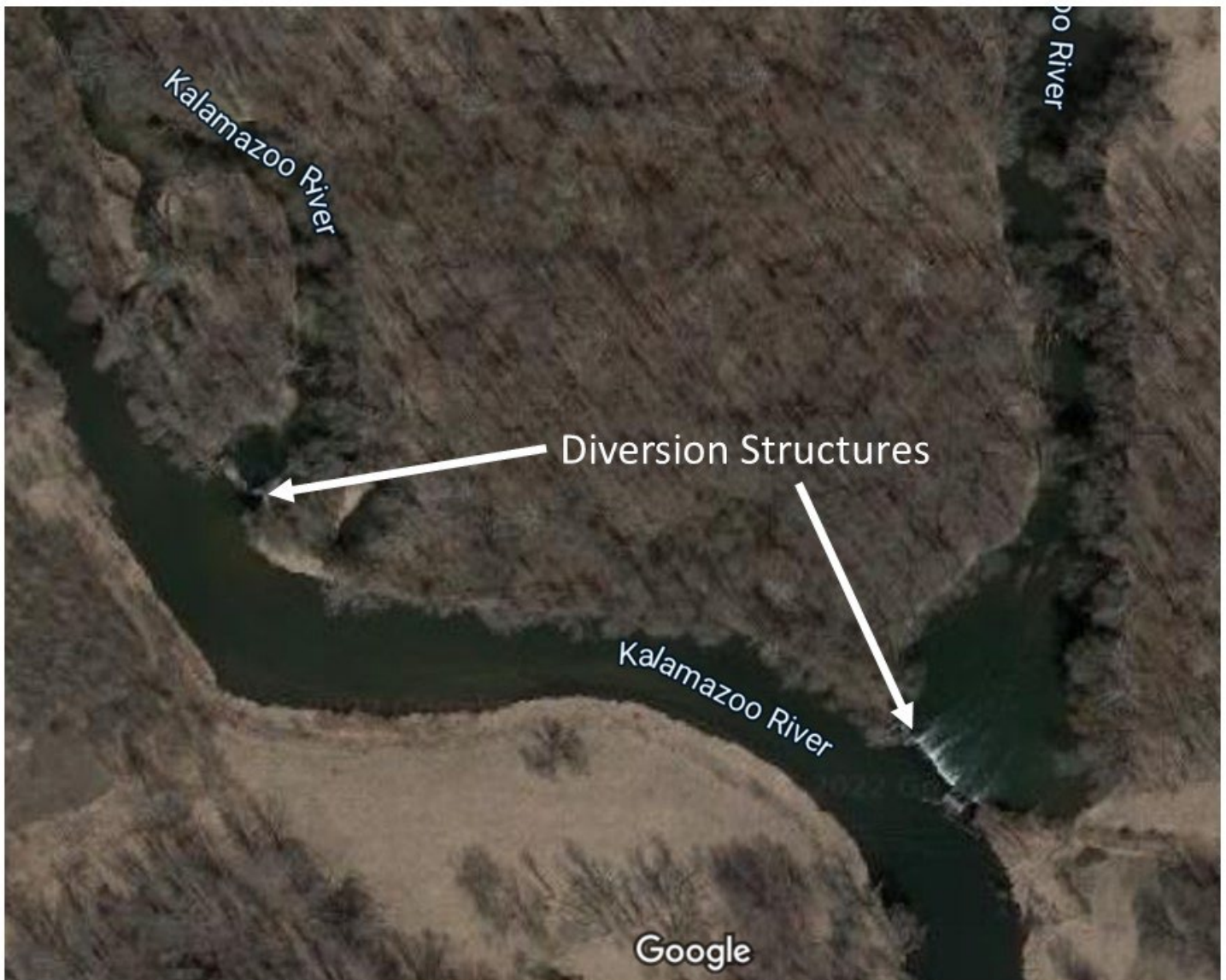
A.3. View of both Diversion Structures – South of City limits
