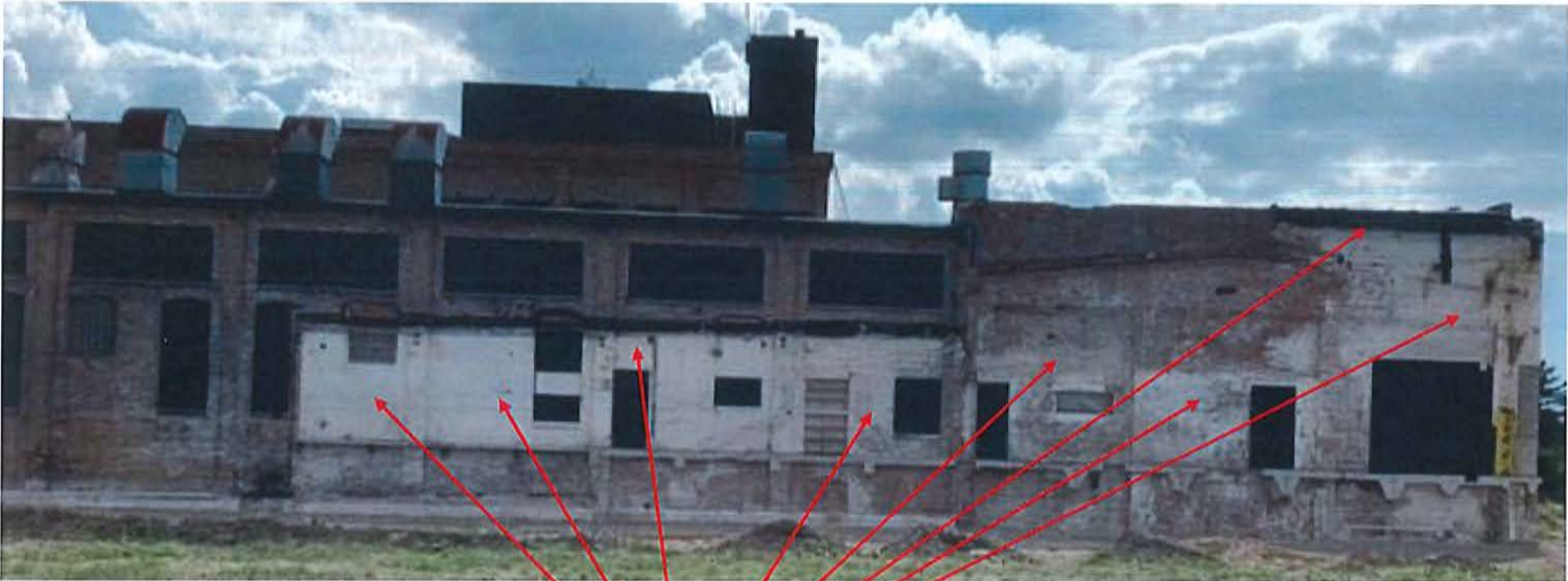
Bld. 10 – West Wall, South End
