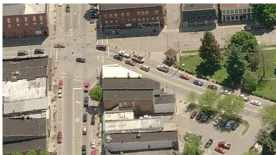
BEFORE: Traffic backup on Allegan Street (looking south) prior to intersection improvements
