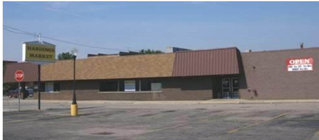
Vacant former Harding's Market, Downtown Plainwell
