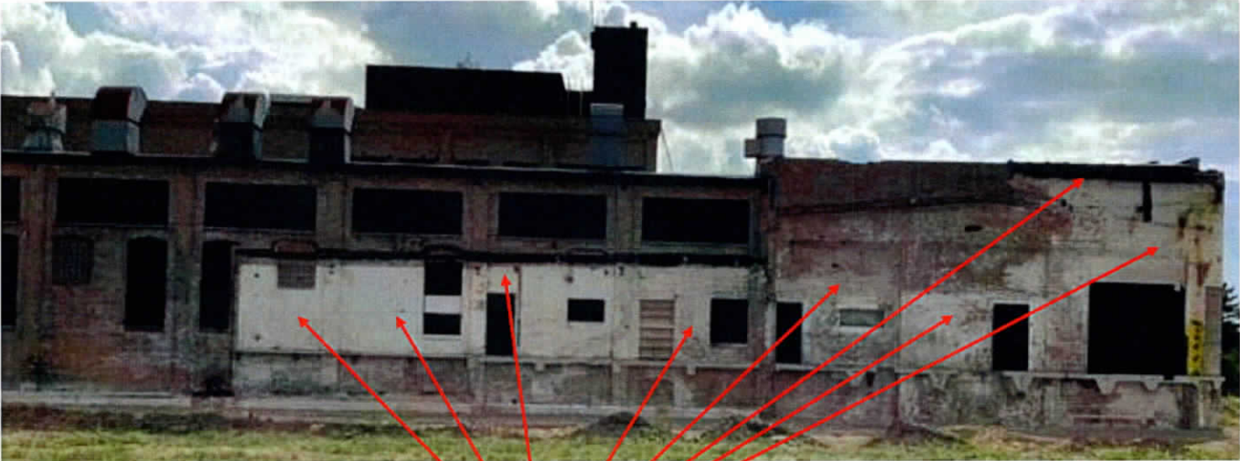
Bld. 10 – West Wall, South End
