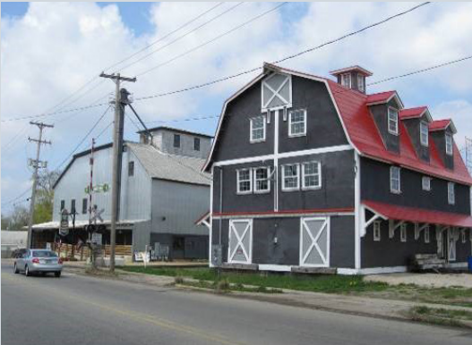
East Bridge Street
