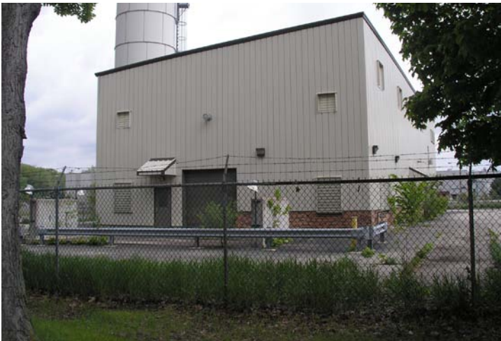
Photo 53: View from the west
