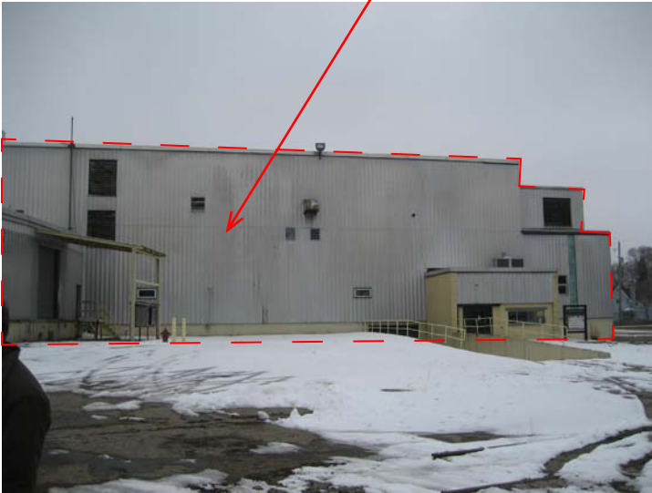
Photo 28: View from the west
