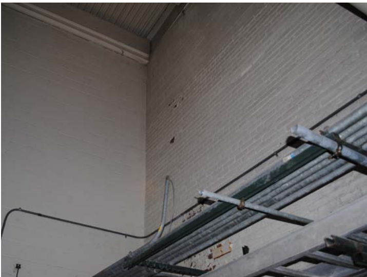
Photo 13: View of seam where buildings are attached
