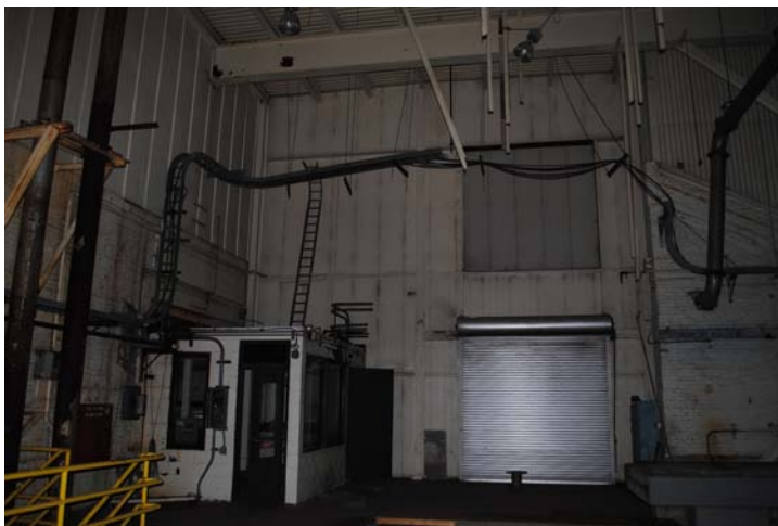
Photo 11: Interior displays a multitude of materials and how the historic building has been modified
