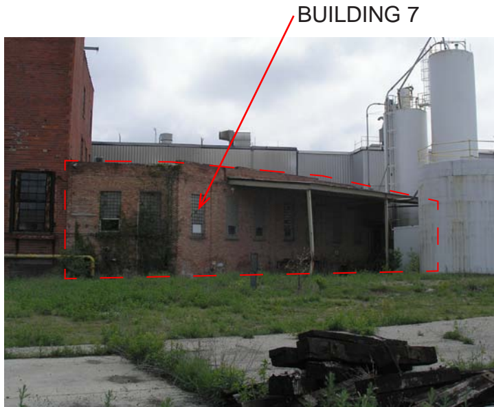
Photo 24: View from the west
