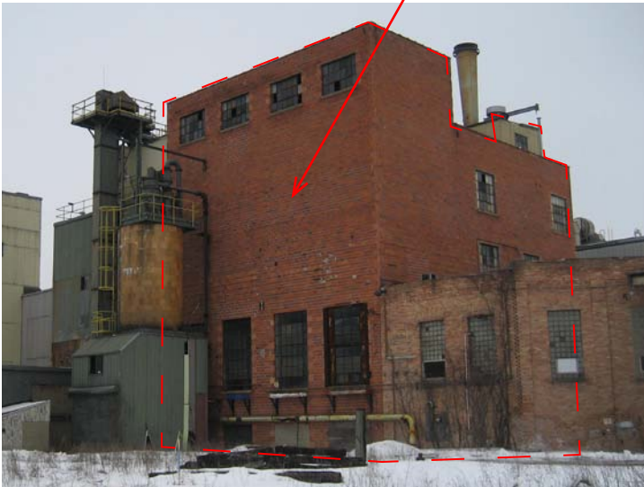
Photo 21: View from the west
