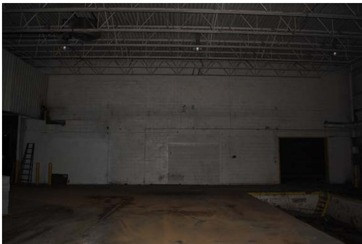
Photo 37: Interior view shows exterior wall of building 16 and connection seams
