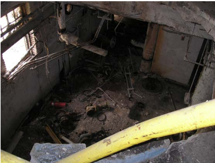
Photo 6: Basement level viewed through a hole where equipment was removed
