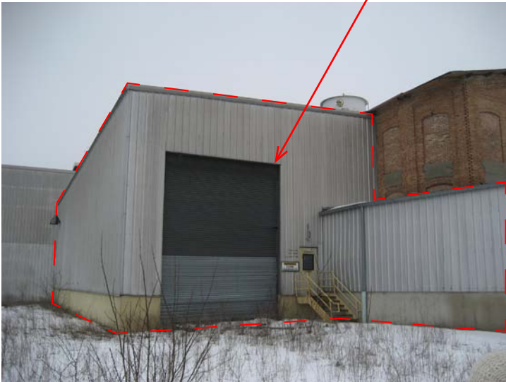
Photo 1: View from south
