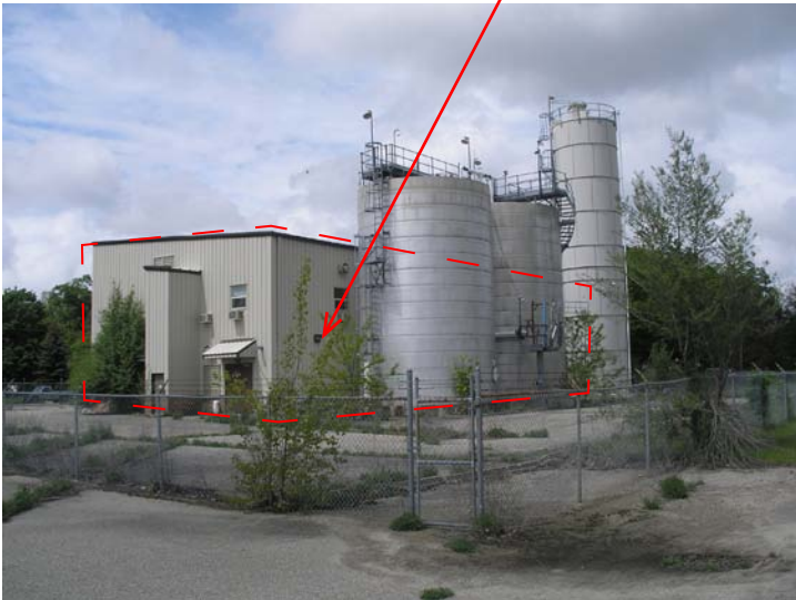
Photo 52: View from the north-east
