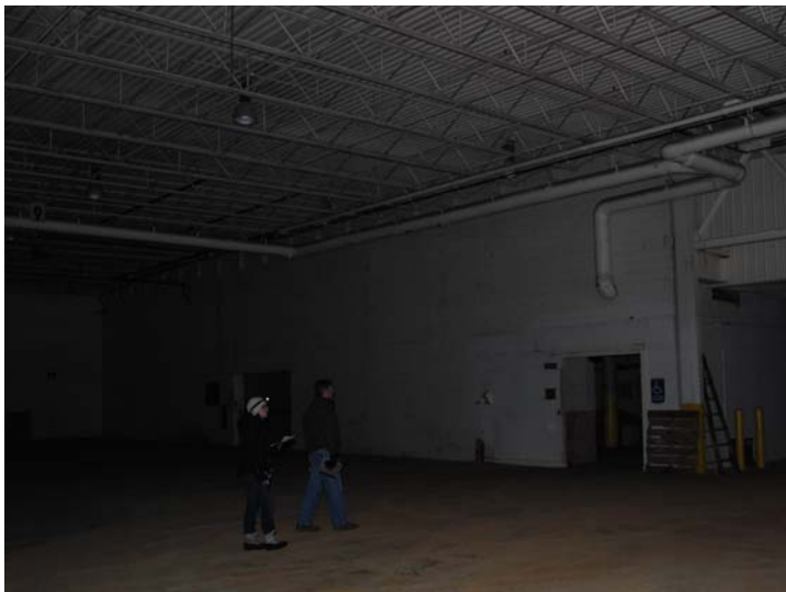
Photo 41: Interior view shows exterior wall of building 23
