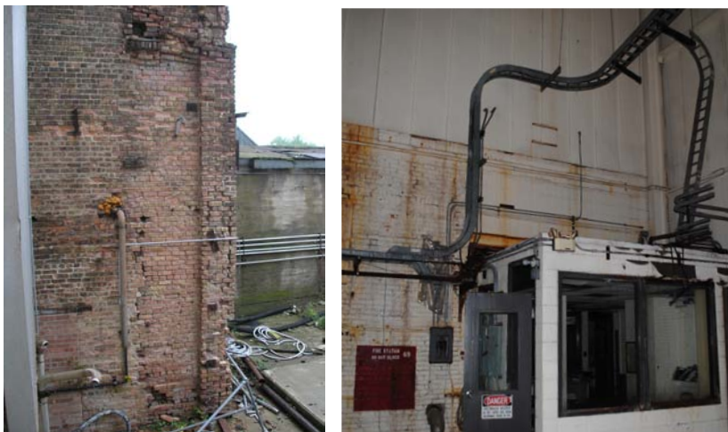
Photo 15 & 16: North-west corner and interior view of exterior wall modifications
