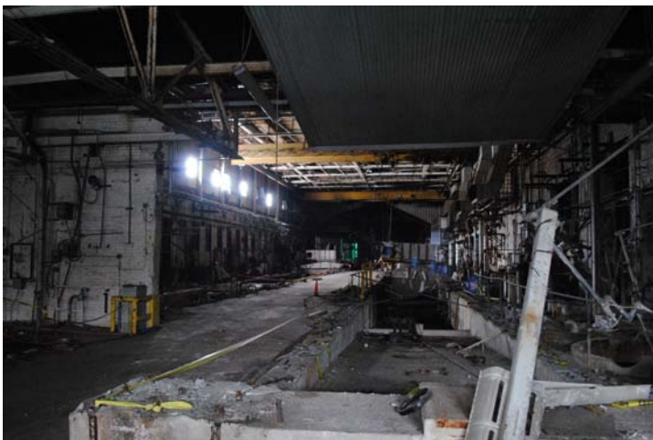
Photo 27: Interior view shows severity of modification
