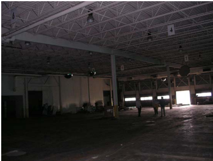
Photo 35: Interior view shows no historic material
