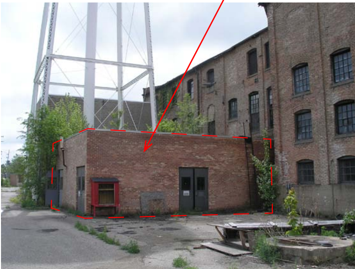
Photo 42: View from the west
