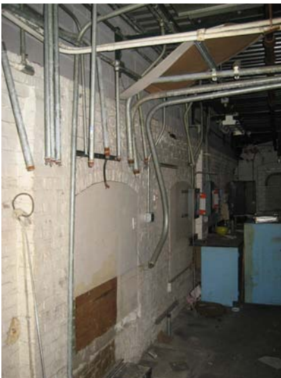
Photo 51: View of the exterior wall of building 4
