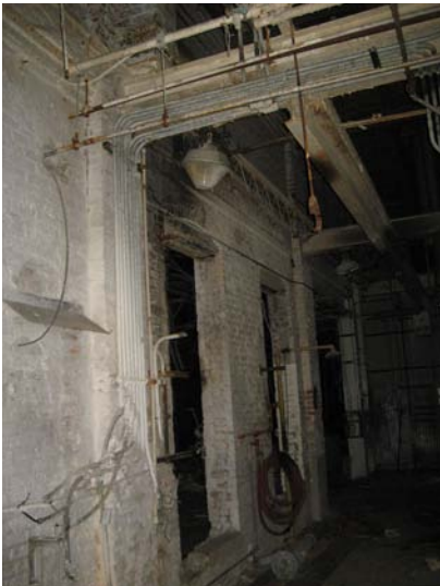
Photo 46: Interior wall of building 10, showing modified fenestration
