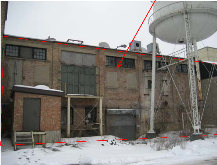
Photo 5: View from north
