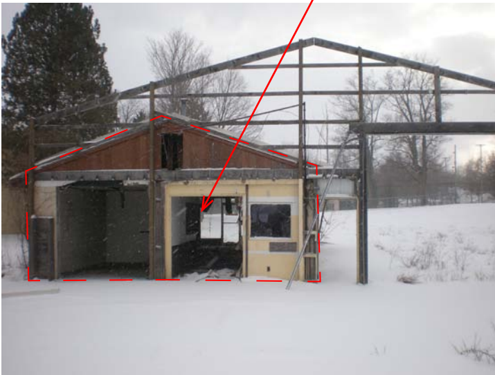
Photo 54: View from the north
