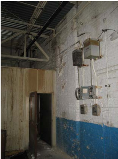
Photo 32: Interior view of building connection
