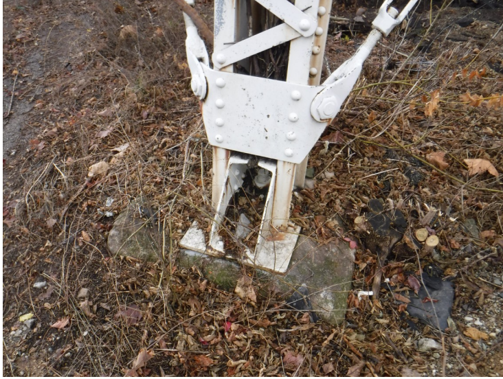
1) Typical leg is in good condition overall. The foundation concrete is in good condition.
