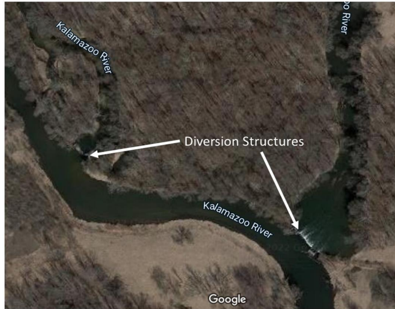
View of both Diversion Structures – South of City limits
