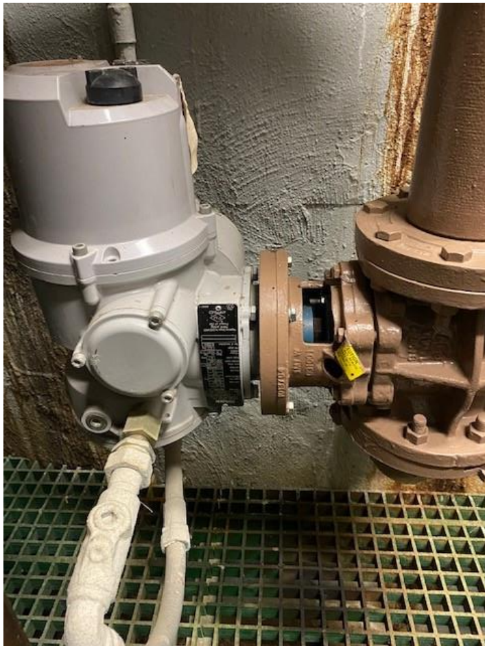
Plug Valve with Automated Actuator
