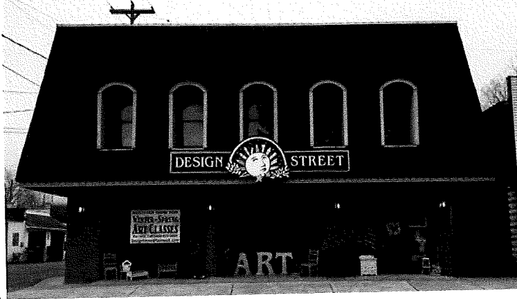
North Elevation (facing West Bridge / Hicks Park / M89)
