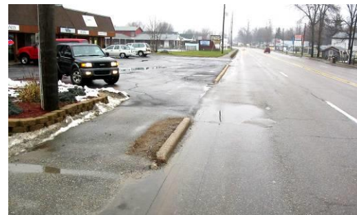
Examples of poor access management. From top: driveway spacing, parking up to pavement, poor driveway definition.
