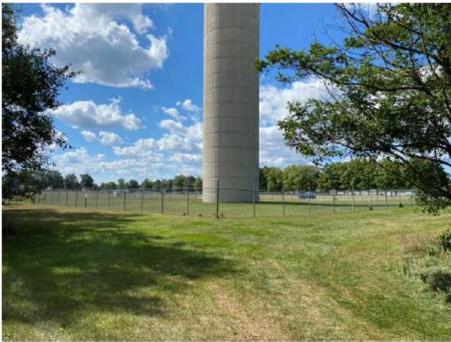
View of Adjacent Property to the West
