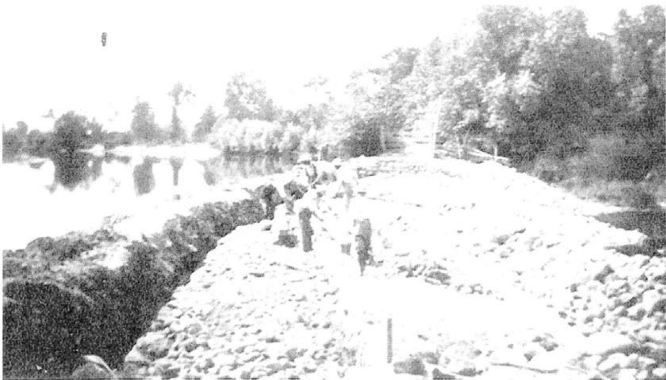
Digging the mill race.
