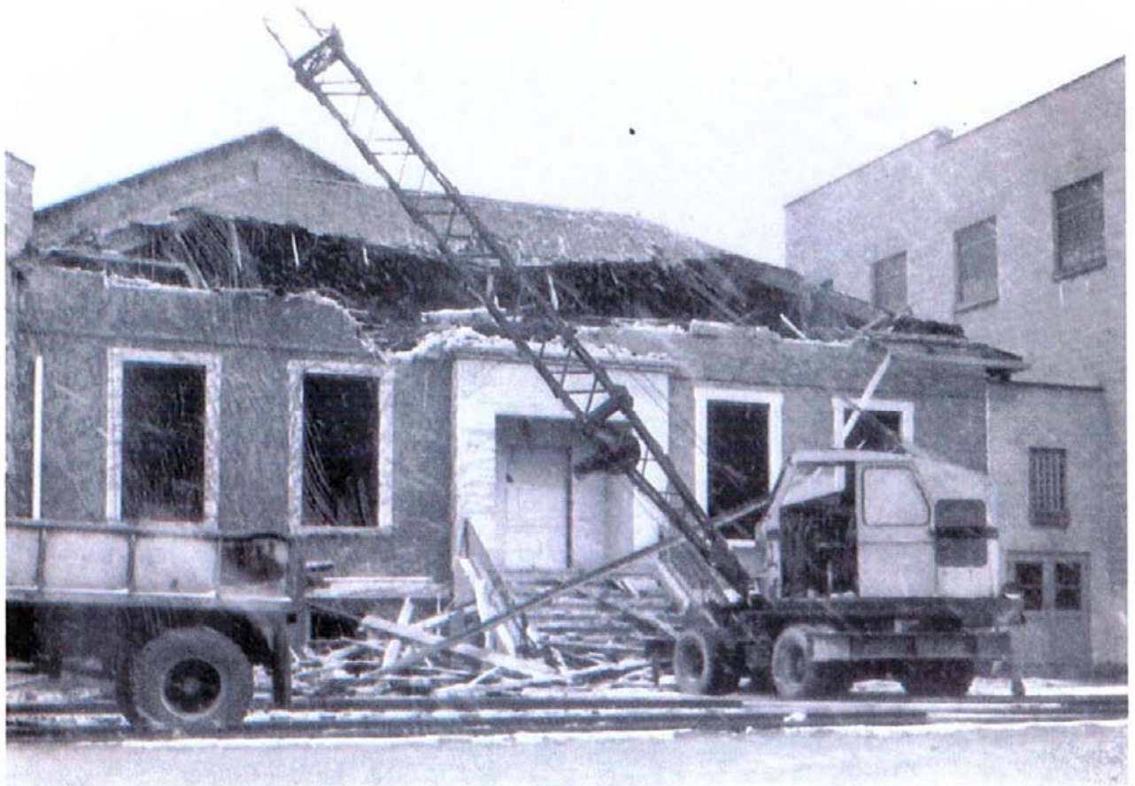
Demolition of several other buildings
