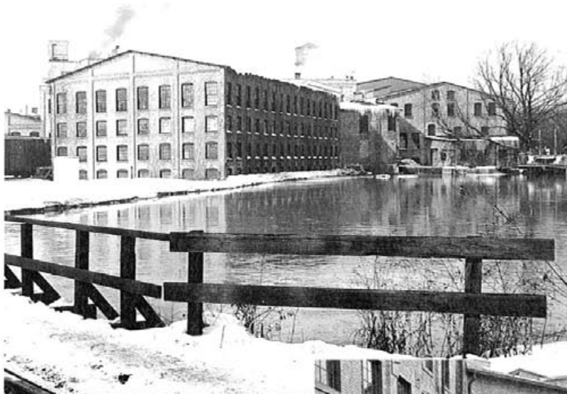
1930's view of the mill shows a wider, higher mill race and evidence of heavier rail traffic
