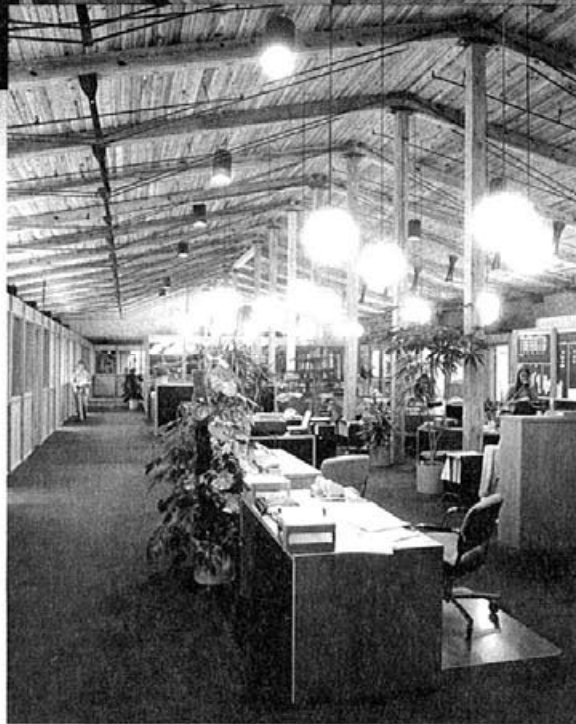
The same area remodeled as the present offices of Plainwell Paper Company. Remodeling was
