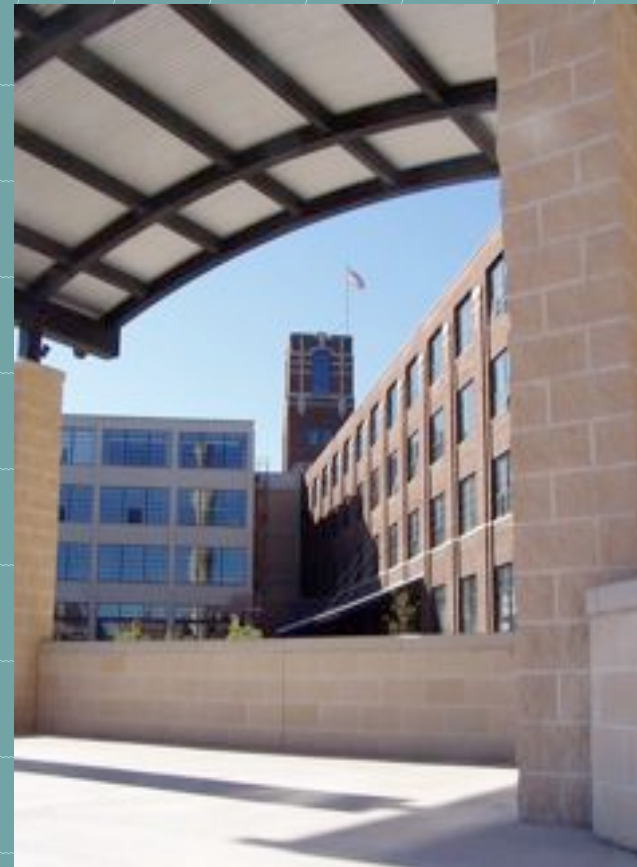
American Seating Co. Building, Grand Rapids
