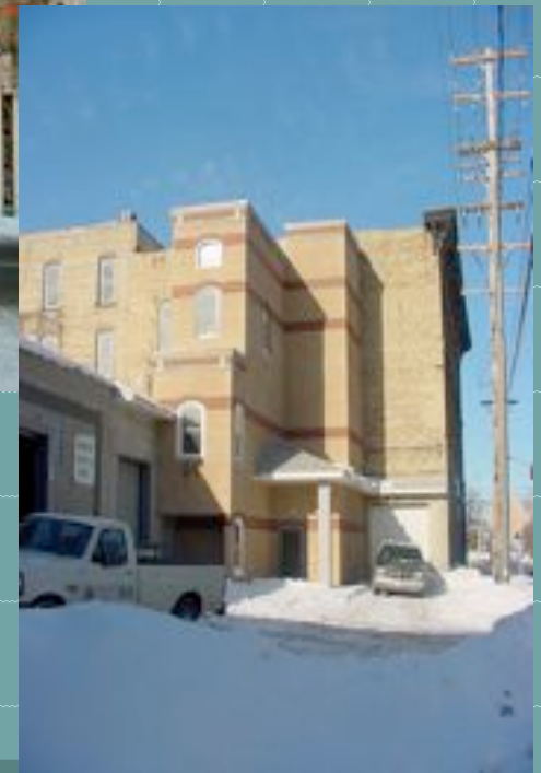
Weirich Building, Grand Rapids
